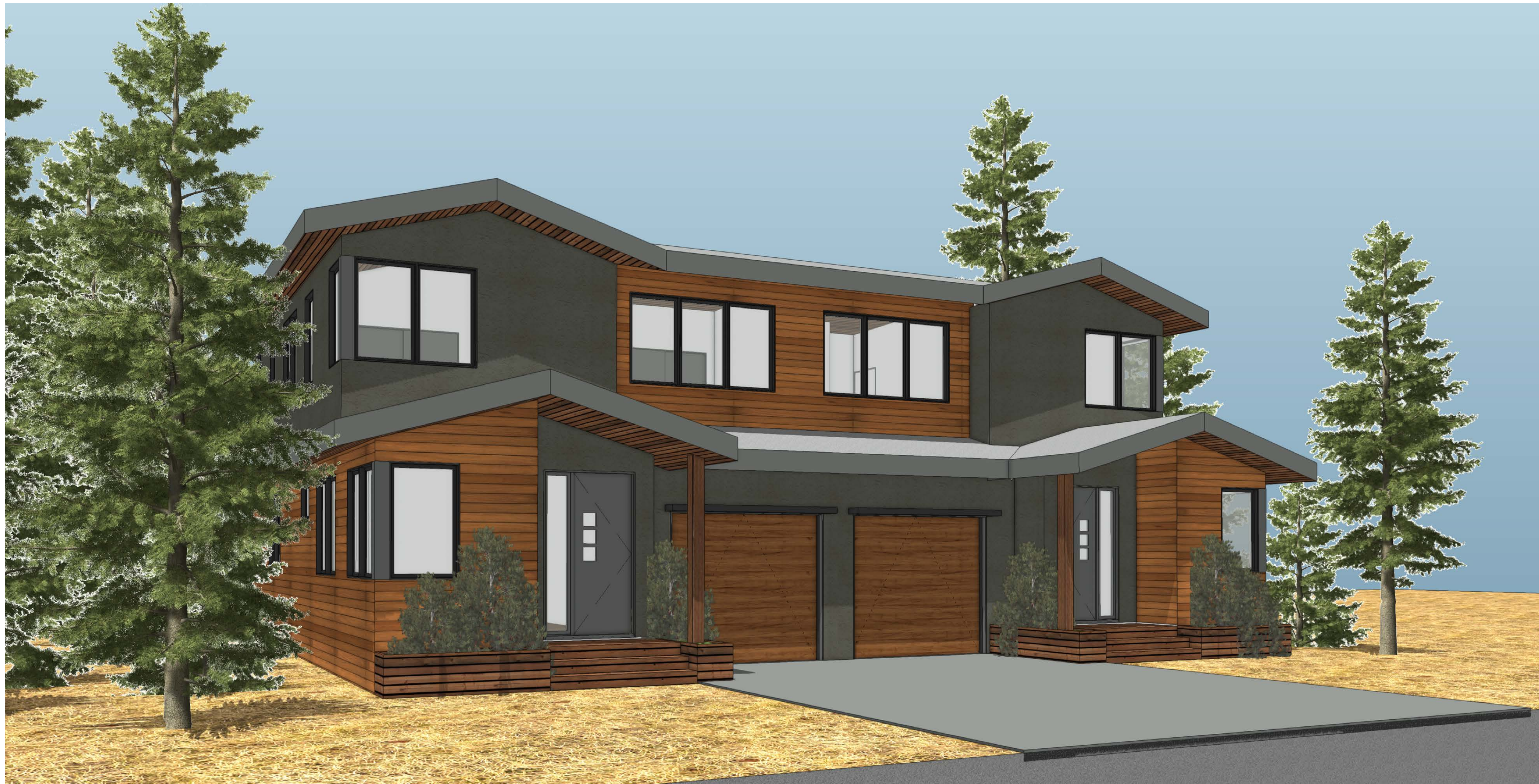
a prefab construction project in truckee, california.
